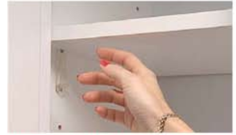
Shelves are 3/4" plywood for improved strength and are adjustable in both base and wall cabinets.
